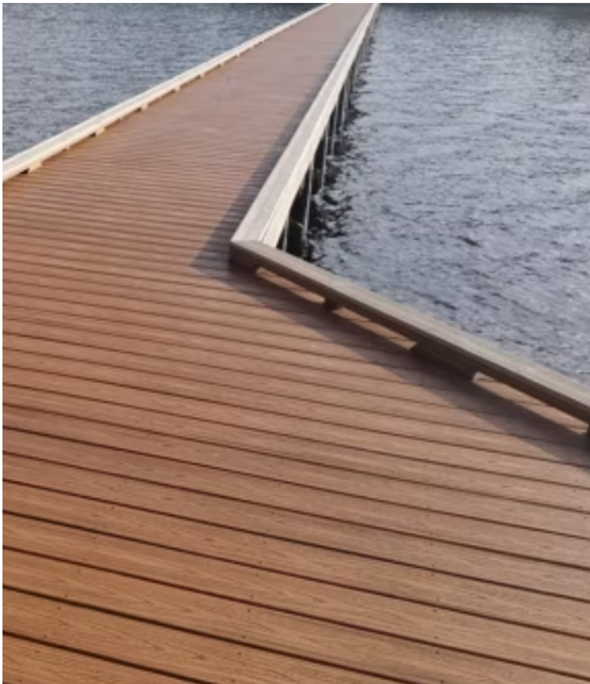
Composite Decking at Fishing Piers
