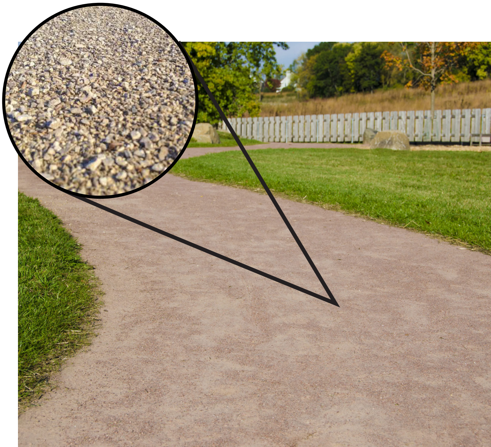
Decomposed Granite Path with Stabilizer Bird Watching Area and Fishing Pier #2 Path
