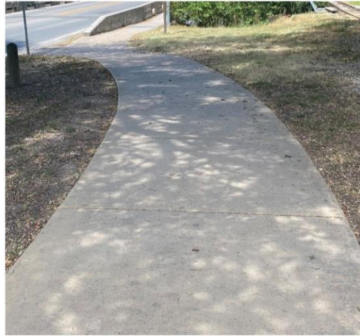
Concrete Pedestrian Trail
