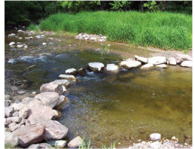
Boulders used as Crossvanes, J Hooks within stream
