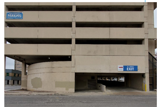
The Wyndham Parking Garage currently exits onto Savings Street.
