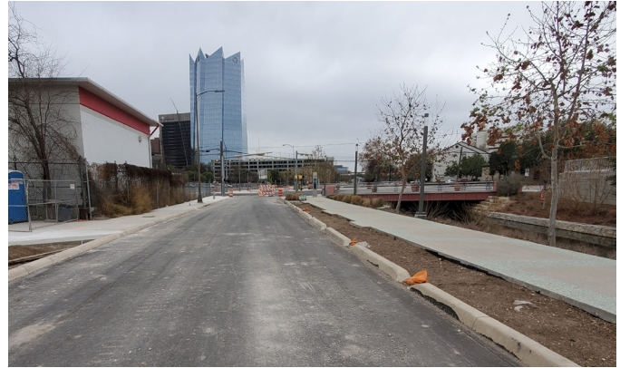
Camaron Street nearing the completion of construction
